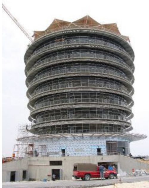
Figure 6. Sakhir Tower in construction.
