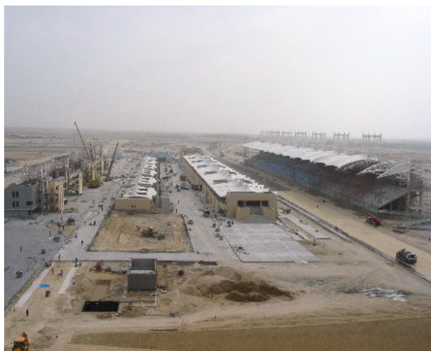
Figure 7. Bahrain FORMULA-1 Circuit project under construction.
